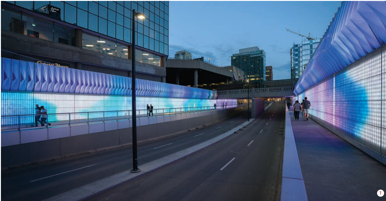
1 4th Street Underpass Enhancement
