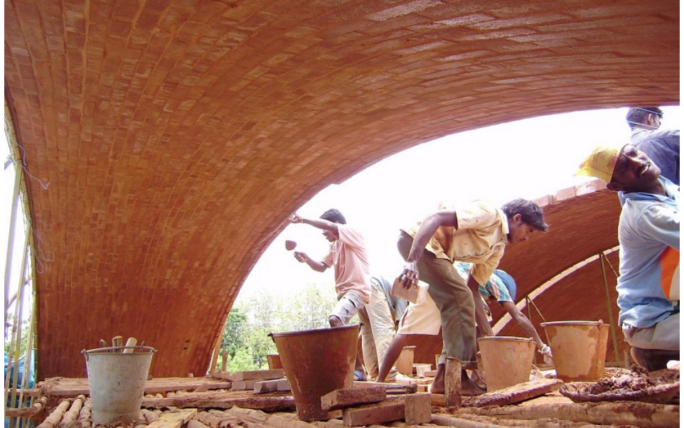
Pondicherry masons constructing a single-wythe 69-meter long by 10-meter wide vault. The earth for these bricks was extracted from a pit on the same site as the building, and the workers were hired by the architect from the nearby village. Internship Jateen Lad Architects/June 2016
