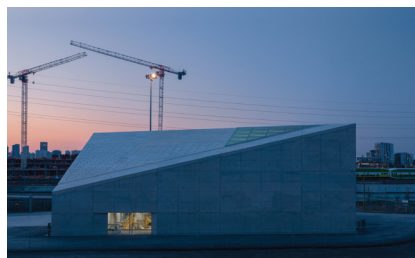
CHERRY STREET STORMWATER FACILITY gh3* R.V. Anderson Associates Limited
