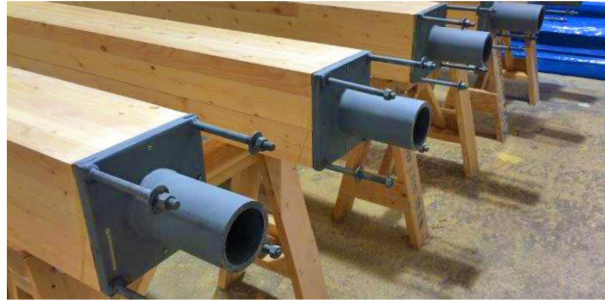
July 2015 glulam columns and steel connectors for mockup
