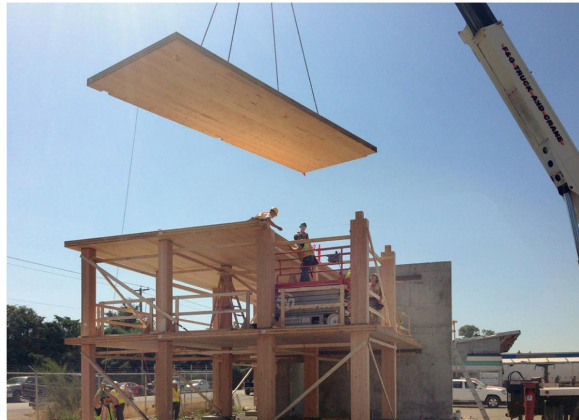
July 2015 erection of mass wood structural mockup
