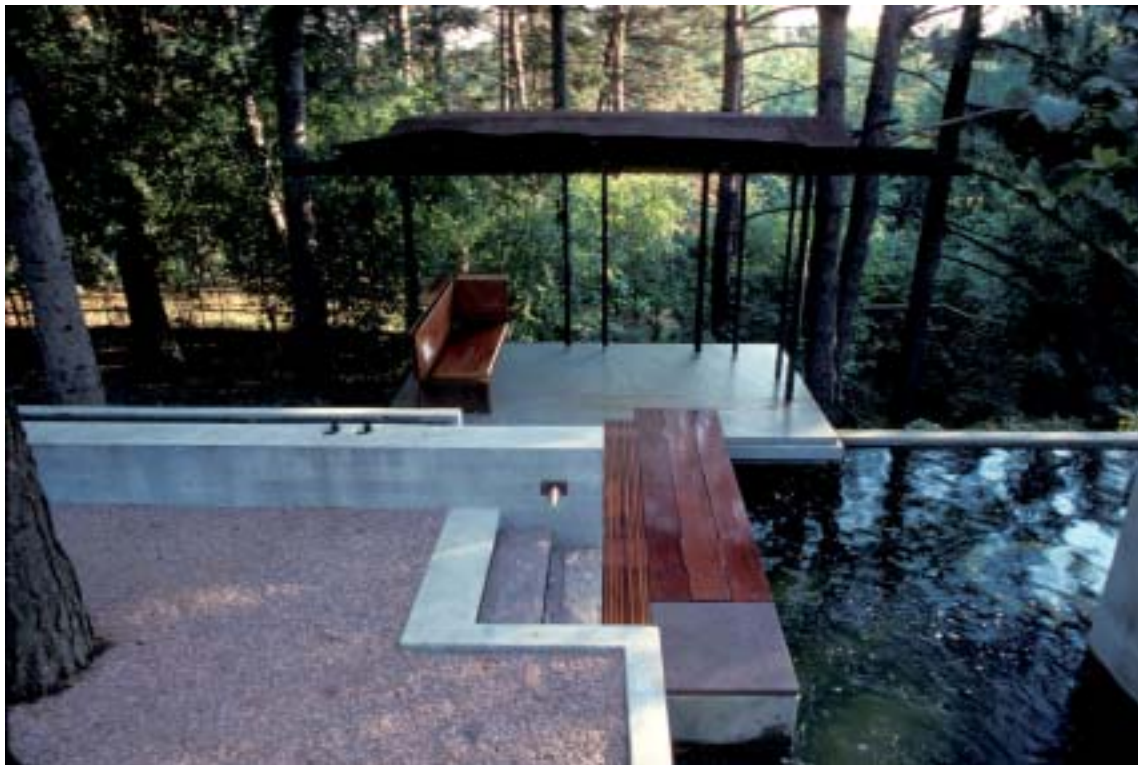
The Frum Garden Pavilion and Reflecting Pool / architecte : Shim + Sutcliffe Architects / photo : James Dow
