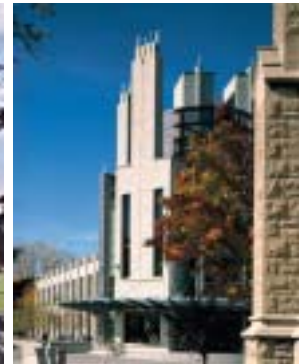
Joseph S. Stauffer Library, Queen's University / architecte : Kuwabara Payne McKenna Blumberg Architects / photo : Jeff Goldberg
