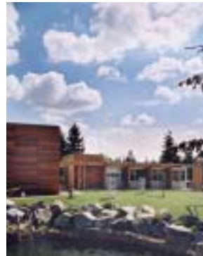
City of White Rock Operations Building / architecte : Busby Perkins + Will Architects / photo : Enrico Dagostini
